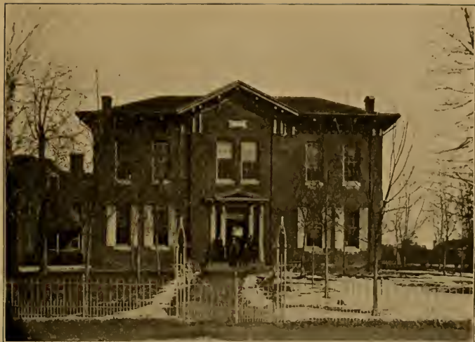
COURT HOUSE AT CHESTERTOWN.
